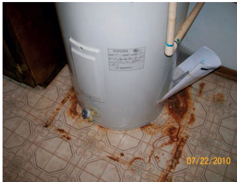
There is no pan installed under the water heater.
